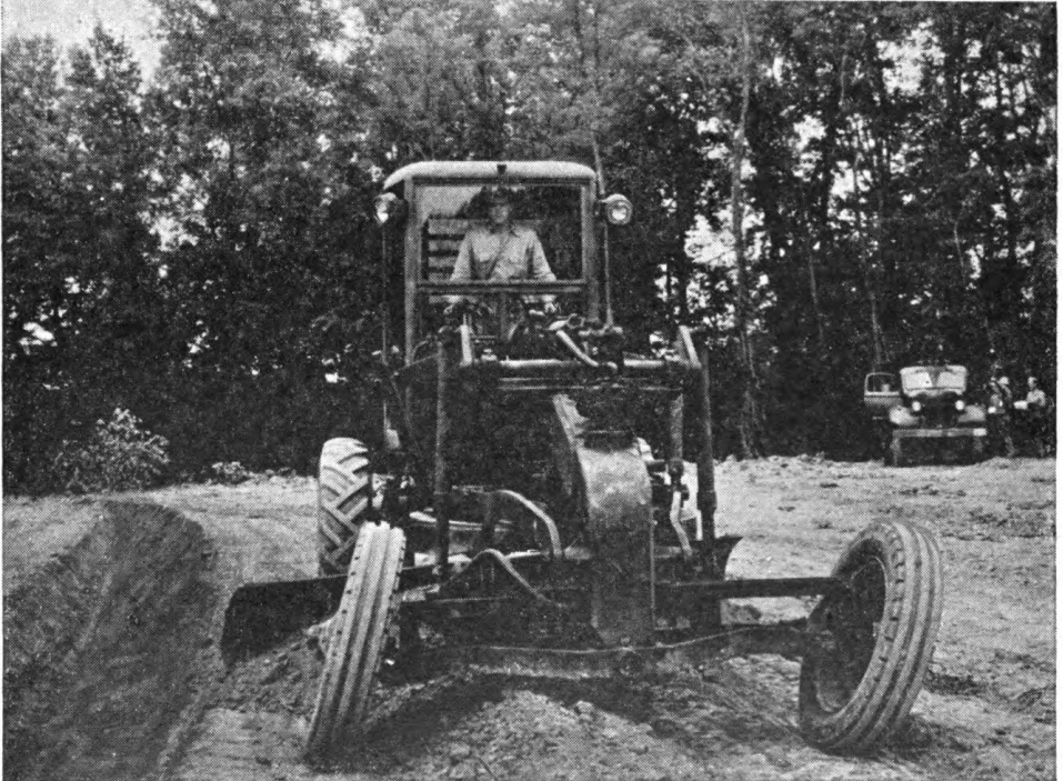
Figure 55. Motor grader cutting open drainage ditch.
